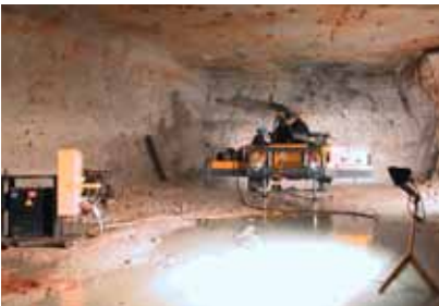
Typical Mining application
