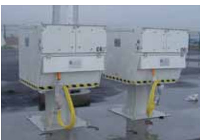
Cavotec Cable Coiler standing 2 x 90kVA
